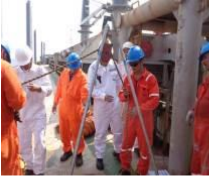
TRIPOD ARRANGEMENT RIGGED USING ROPES AND BLOCKS
