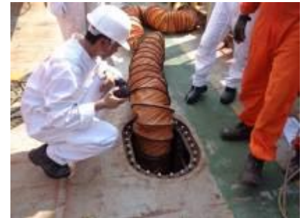
ADDITIONAL VENTILATION PROVIDED
